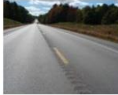
2-Lane Roads 80-90km/h (Milled rumble strips)
