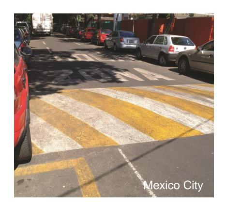
Speed humps are simple but effective ways to lower speeds. Newly installed humps have shown to reduce mean vehicle speeds from 36.4 to a designed speed of 24.4 km/hr.
